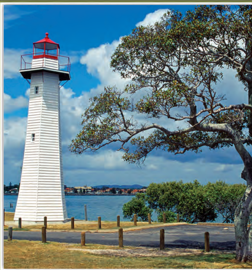
QLD - LIGHTHOUSE AT CLEVELAND
